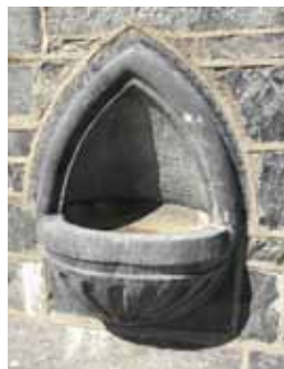
One of two inset carved limestone water fonts left and right of the entrance arch to St Nicholas' Church.
